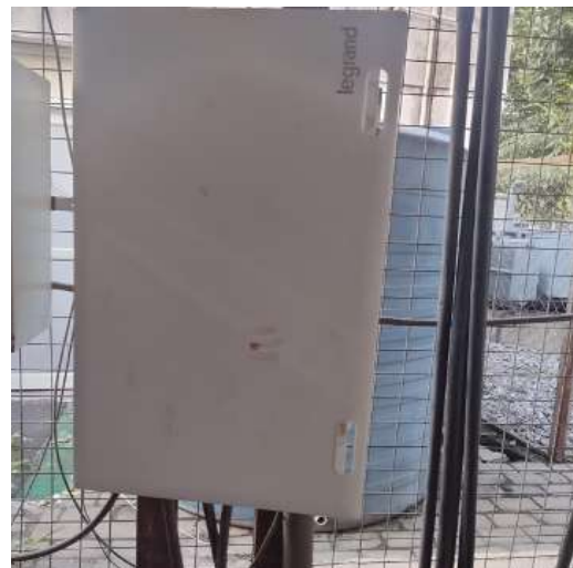
DB without identification and Danger notice DB support frame is corroded
