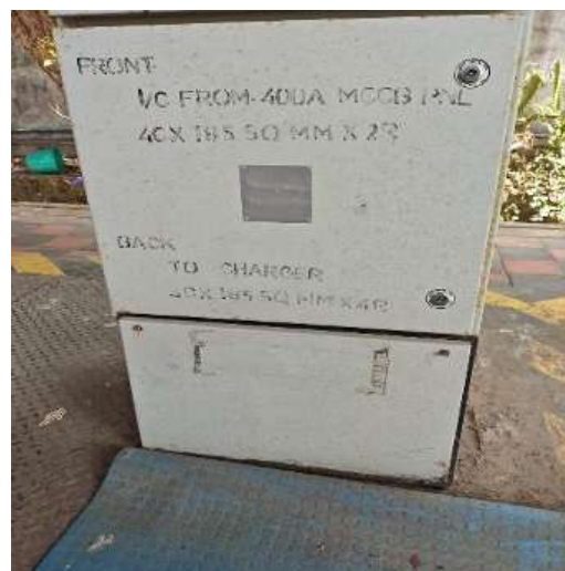
Protective rubber mats in front of DB
