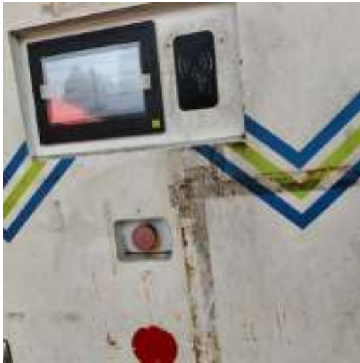
No identification label for Emergency PB
