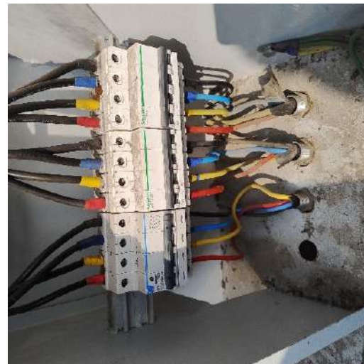
Unsealed cable entry, No ferrules, Missing door earthing
