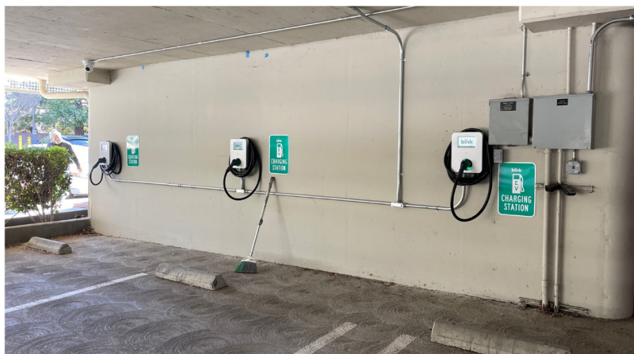
Figure 8 Installed EV charging station at GHS A
