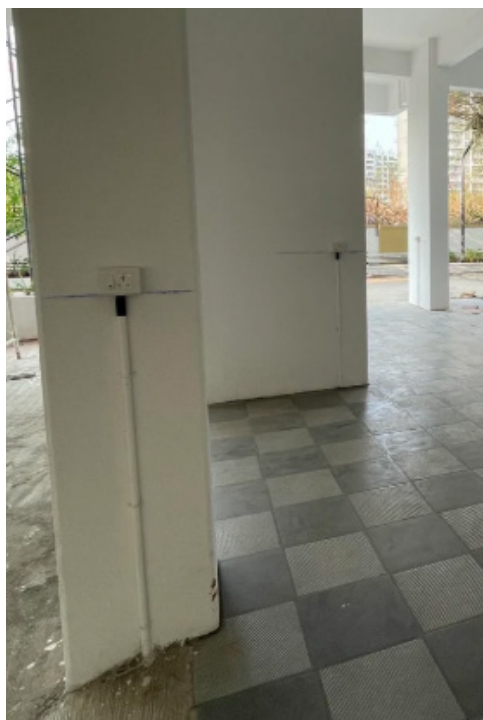
Figure 11 Individual stilt parking in Pune, Maharashtra with 16 A provision for EV charging
