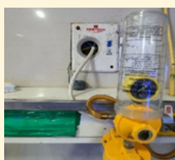
SNCU Area (cable insertion without socket)
