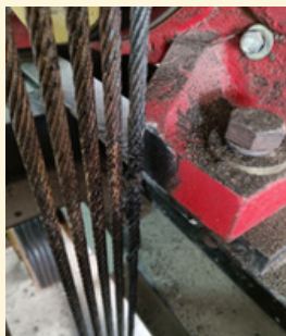
OPD Lift Area (Wear & Tear of ropes)
