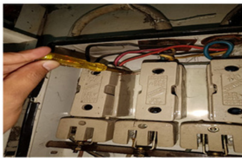
FF Children Specialist DB (Fuse is bypassed here with bare conductor which was found live)
