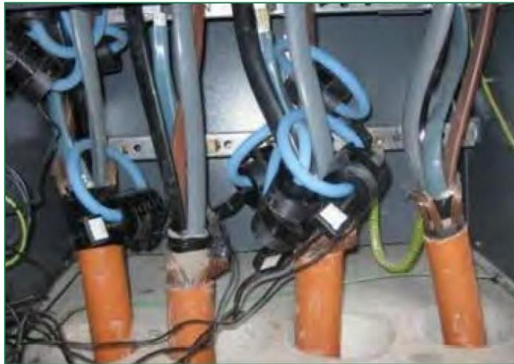
**Figure 4: Installing Rogowski sensors (blue color) for PQ monitoring**
