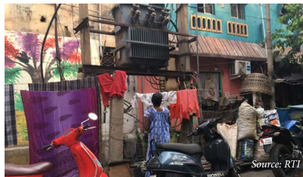
b) Illegal Occupancy in port area
