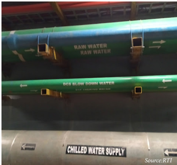
Figure 6.7: Underground Utility Tunnel in GIFT city
