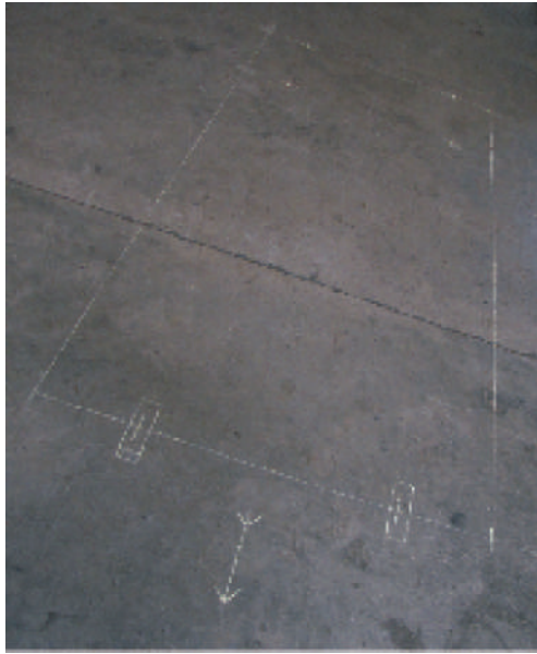
b. Marking the system layout with chalk on the terrace.
