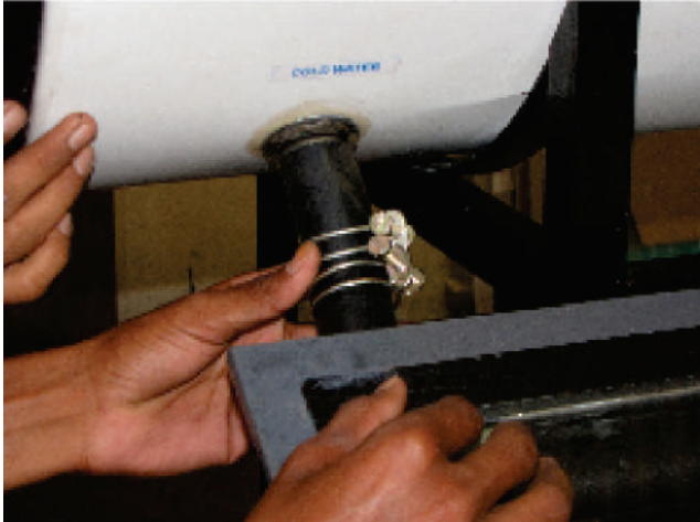
f. Connection between collectors and tank ( hose/system piping)
