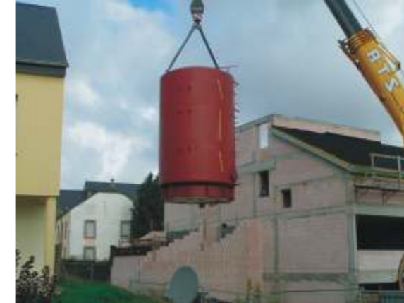
Fig 11: Installation of storage tank
